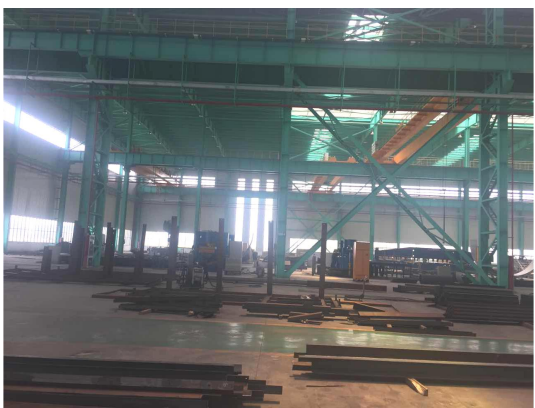
探伤铅房拟建址北侧
